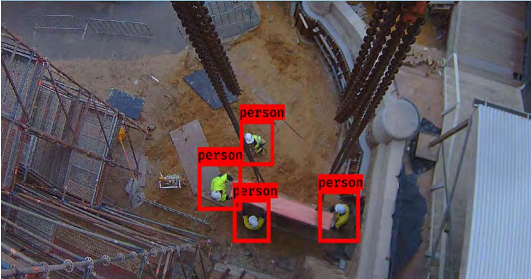
Roborigger is developing a personnel detection system based on an artificial intelligence (AI) model to **detect personnel within the fall zone** of a suspended load. The prototype system is already working.
